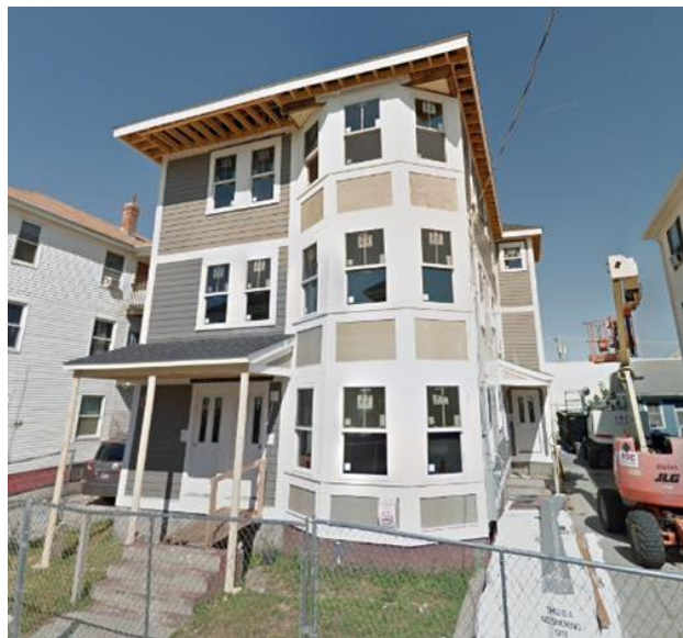
Knight Street House, Pawtucket, RI – "Branch Street Revival"
