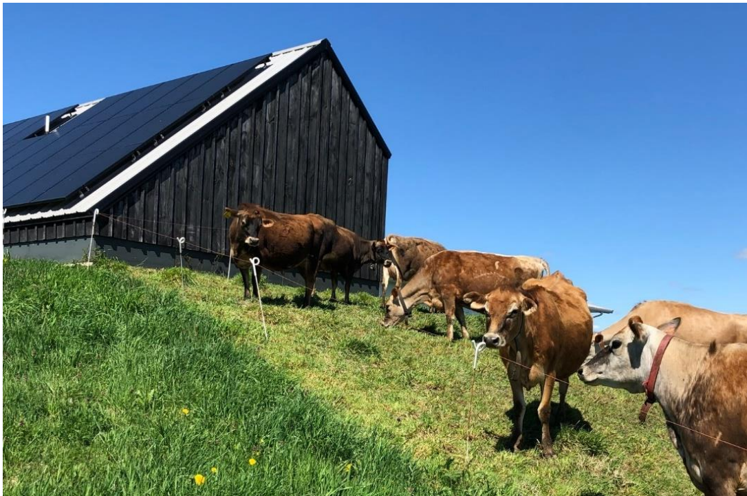
Figure 1: Rooftop Solar array at Sweet & Salty Farm, Little Compton, RI RIAgEP, REAP, and the Renewable Energy Fund were all used to fund this project
