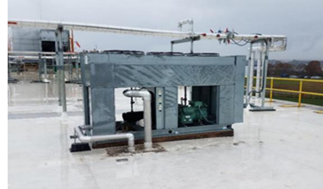
Rooftop condenser and compressors packaged in one unit
