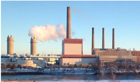
Increase power production
