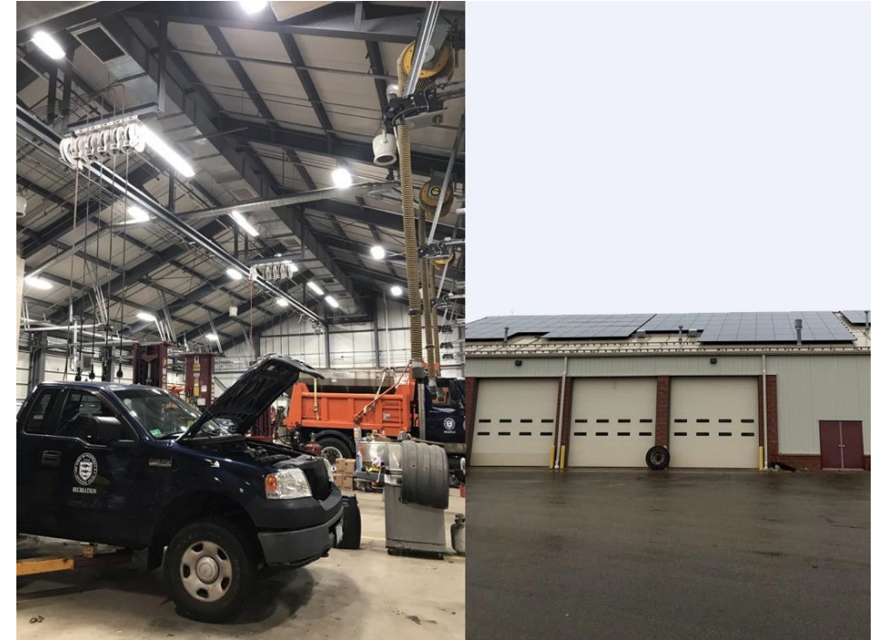
Town of Westerly Public Works Facility
