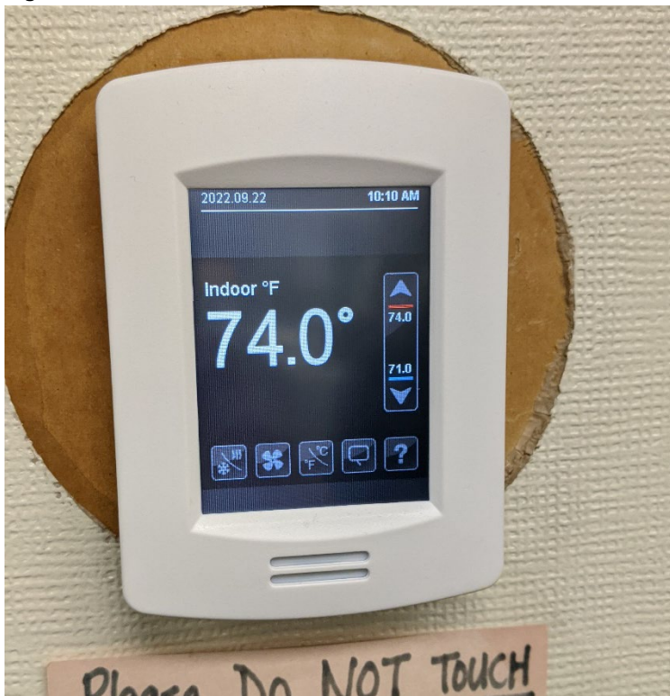
Figure 1-2. Zone 2 back office Wi-Fi thermostat
