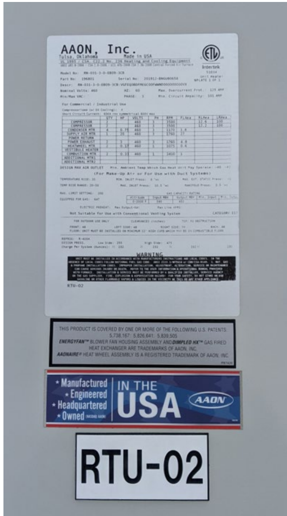
Photo 2-1 Nameplate RTU-2
