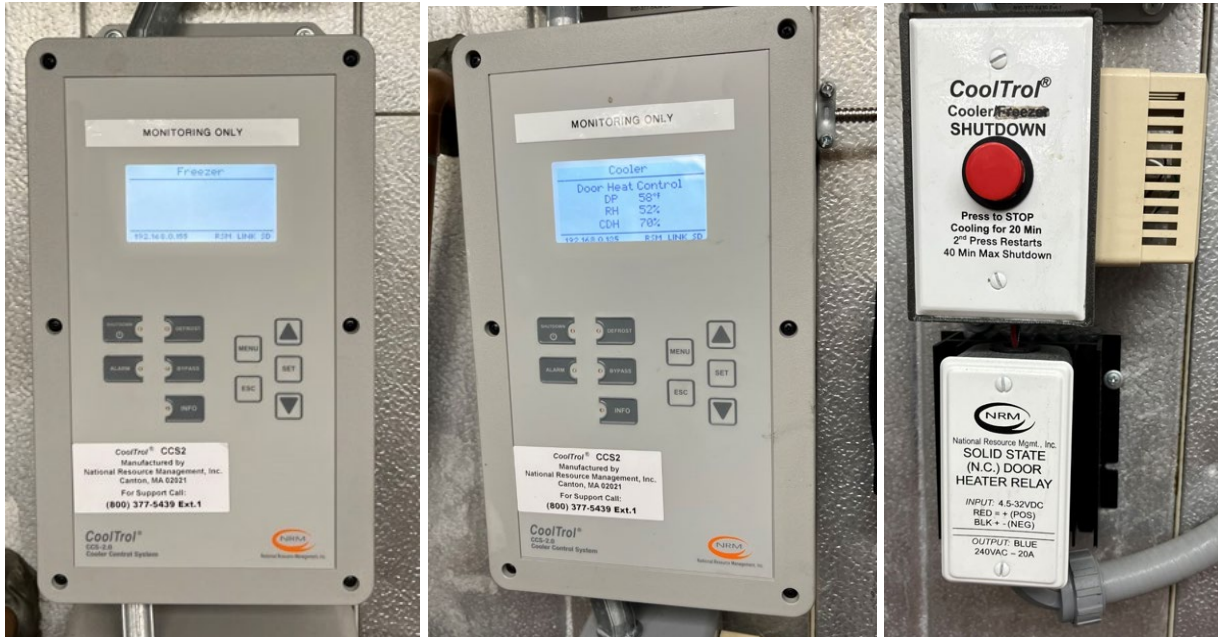
Figure 2-9. Walk-in Controllers
