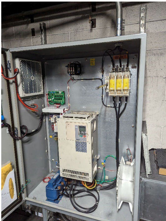
Figure 2-3. Dust collector panel and VFD
