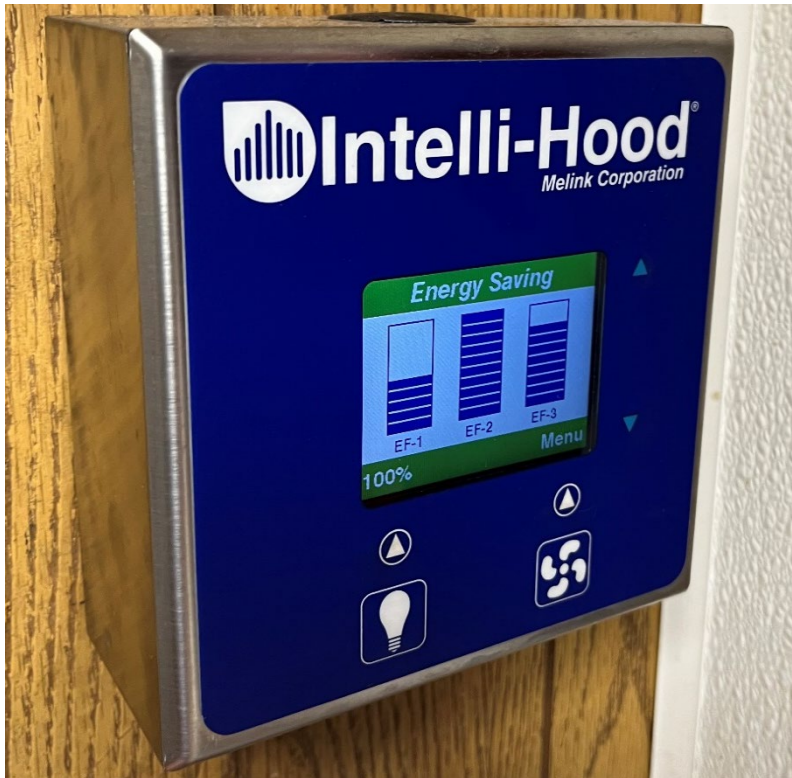
Figure 2-7. Kitchen Exhaust Fan Controller
