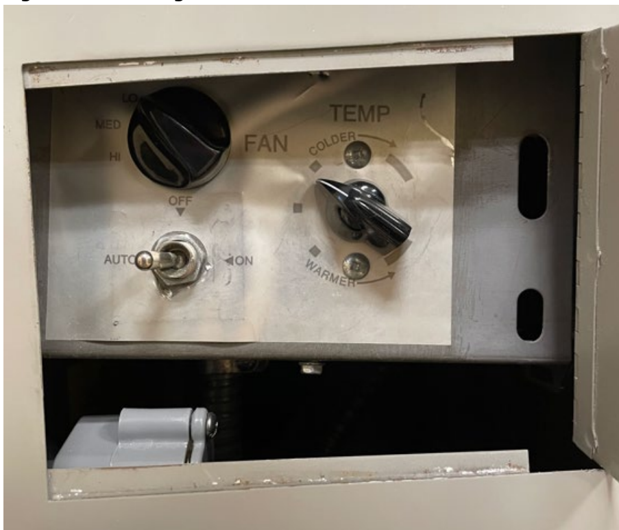
Figure 2-6. Existing Case FCU controls
