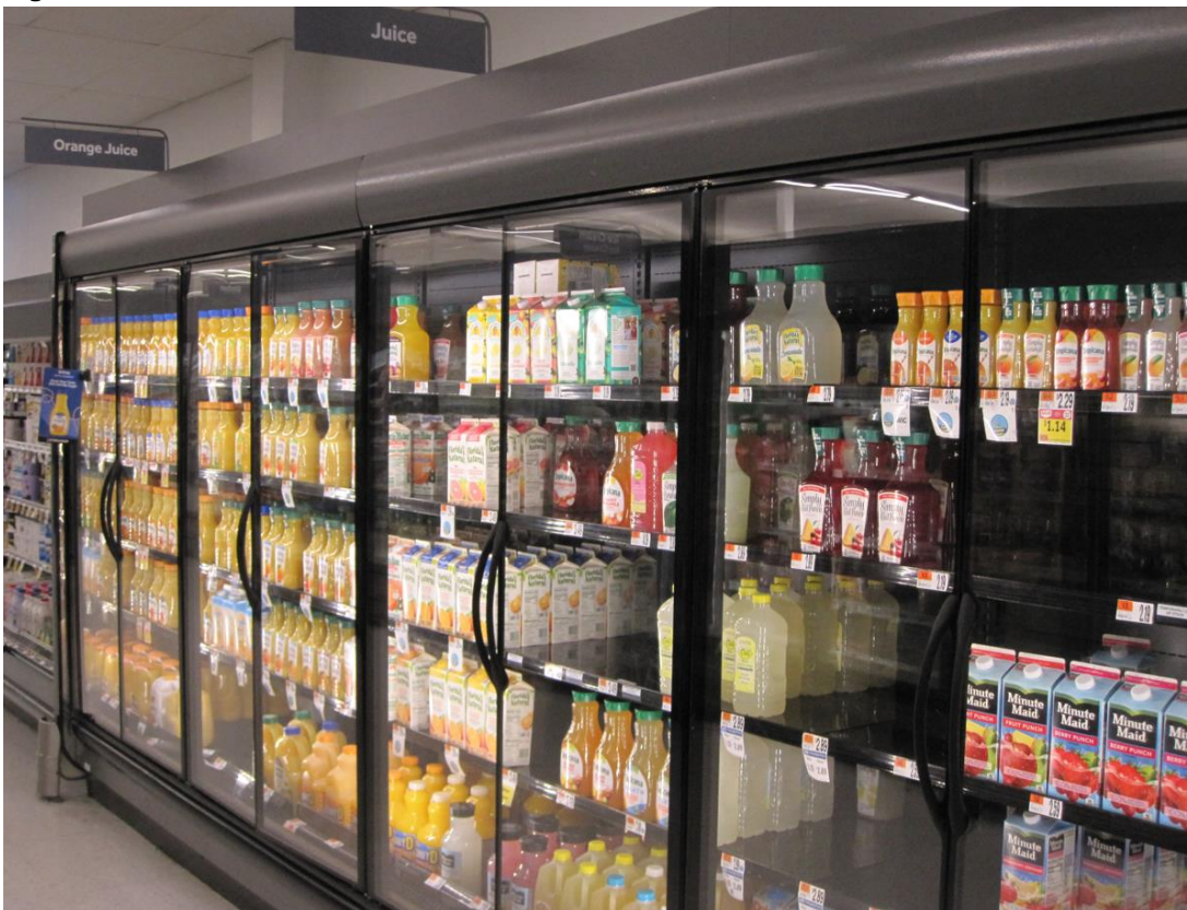
Figure 2-6 Installed case doors
